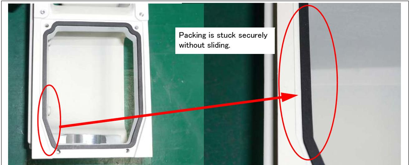
Fig.5-5 : Example of sticking packing (good example)
